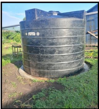
Two tanks, each with a 10,000 litre capacity, were purchased to help harvest water from the heavy rains.
